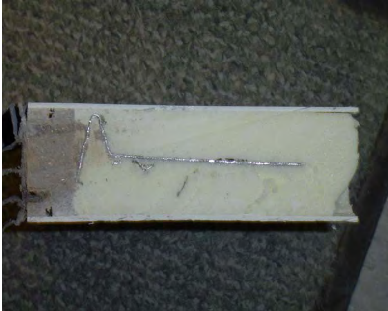
Leaf Cross Section at Bottom Rail
