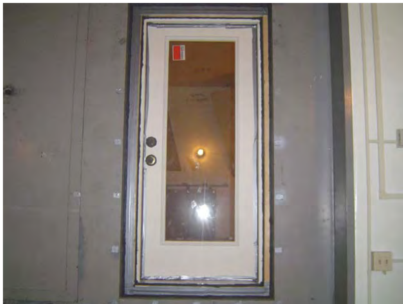
Source Room View of Installed Specimen (Inoperable)
